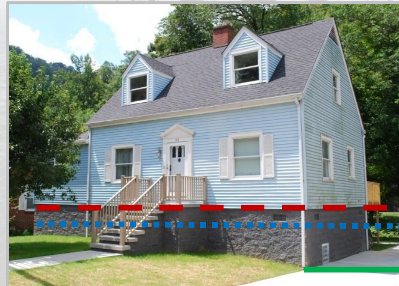
Residential structure post-elevation
