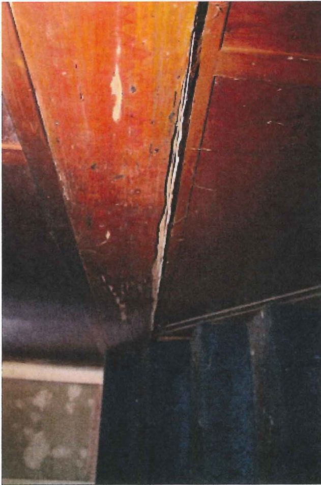
21. The staircase is not stable and the staircase walls have separated. (picture 21)
