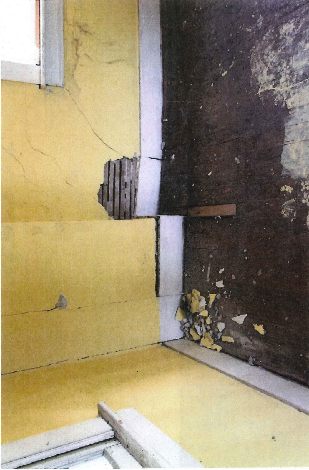
18. The upstairs bedrooms are not level. Both rooms are leaning to the left. (picture 8b)
