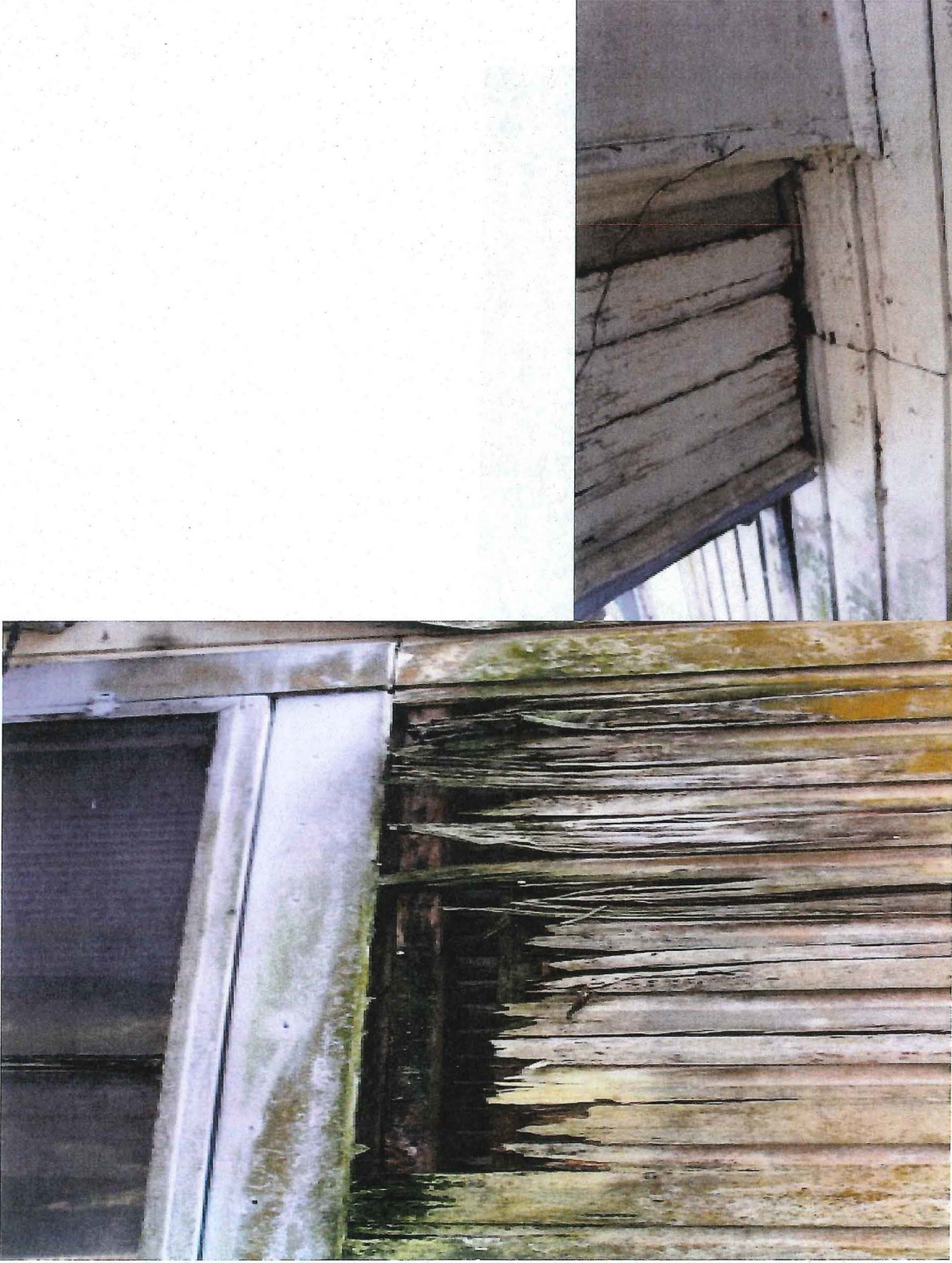
6. The exterior wood and supporting beams have significant water damage and wood rot. (pictures 6-6a)
