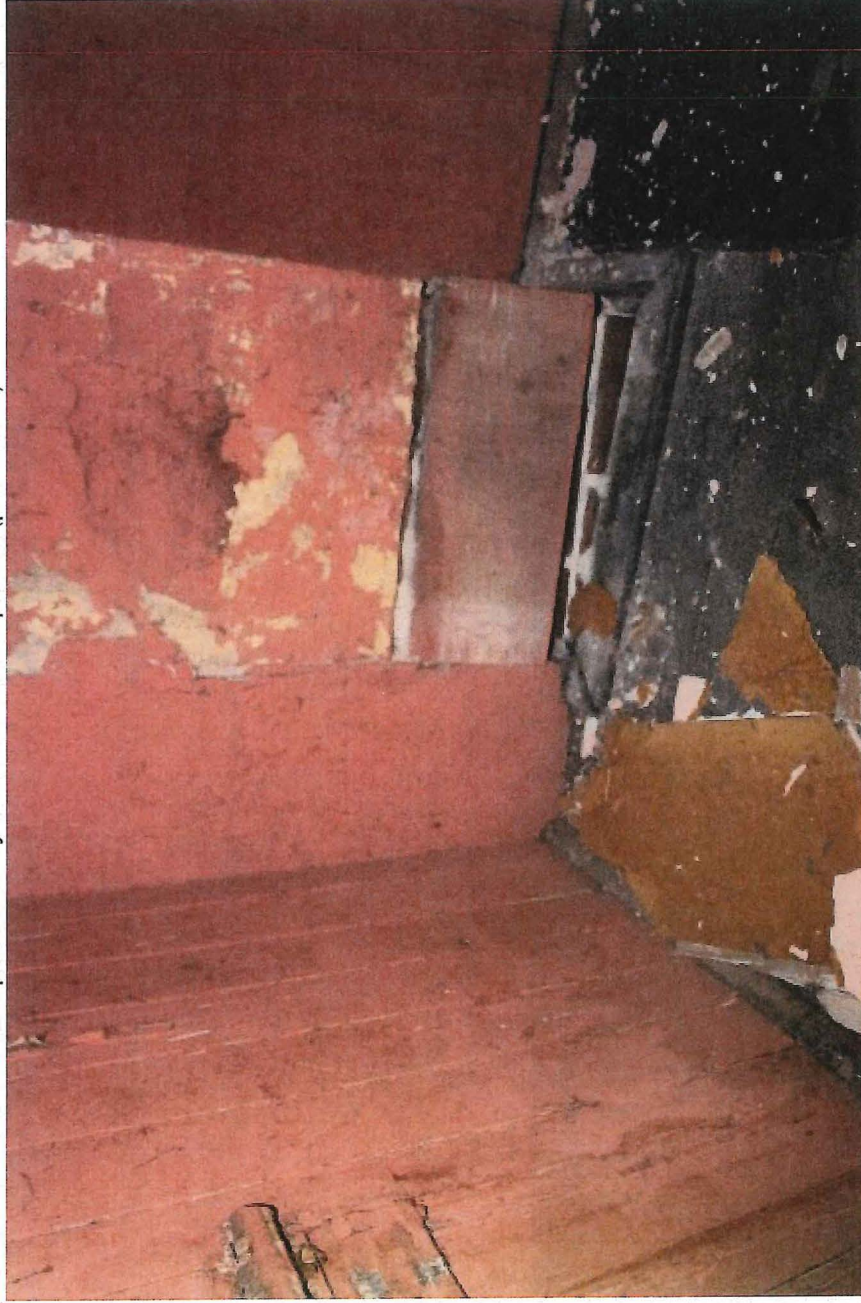
20. The floor is slanted and pulled away from the old fireplace. (picture 20)
